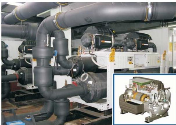
**Figure 1. New water chillers with TurboCor compressors**
